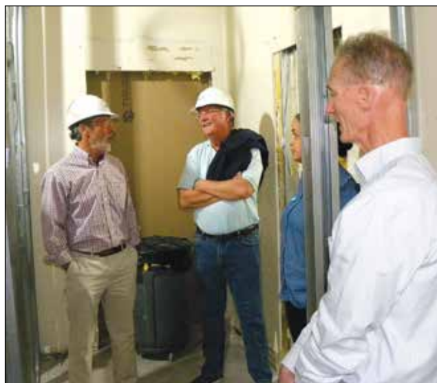
Lawrence YMCA Building Committee Chair Tom Childs tours the new pool viewing area with Merrimack Valley YMCA Board of Directors member Greg Schmidt, Membership Coordinator Rocio Diaz and Project Manager Rick Feldman.
